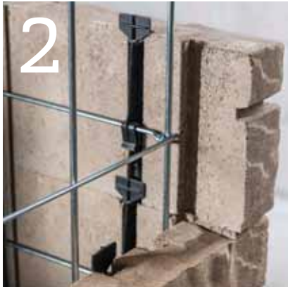
Use connector to attach Tandem Units to grid
